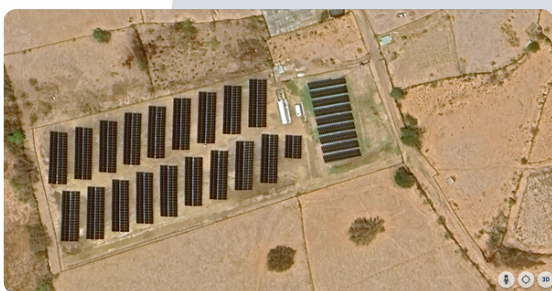
Limlair Facility Pre Hurricane Beryl
