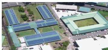
Aerial view of TAMCC's solar energy installation.
